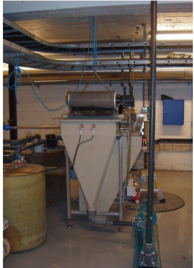
Figure 6: Sludge filter that takes the fine particles out of the condensate.
